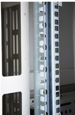
19" profiles marked with U height position
