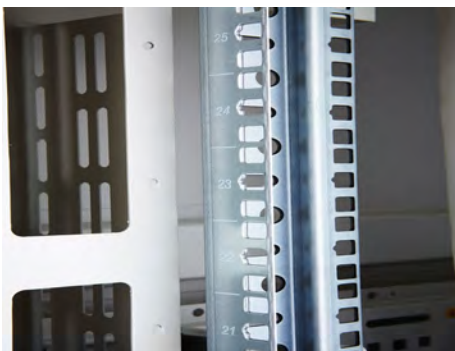
19" profiles marked with U height position
