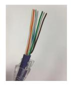
Straighten all 8 wires as shown
